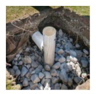
**Soak away (or soak pit):** is essentially a pit designed with the purpose of allowing treated wastewater to infiltrate into the ground. A soak pit should be located more than 50m from drinking water sources (e.g. Boreholes), and never less than 2m above the groundwater table.
