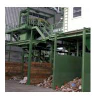
**Transfer station:** is a larger, formal waste transfer facility where waste is brought in, often processed somehow (e.g. sorted and/or compressed). When a sufficient amount of waste has accumulated at the transfer station, this waste can be removed and transported to a waste reduction facility or to the final landfill site.
