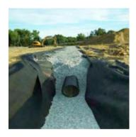
**French drain:** is a trench that is filled with gravel, which then acts as a conduit for water runoff. A common design for a French drain might include a perforated drainage pipe wrapped with filter cloth/membrane, submerged in course aggregate (gravel) and sloped for drainage.
